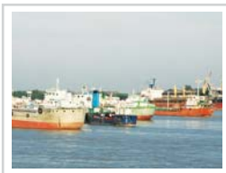
Partial view of the Chittagong Port
